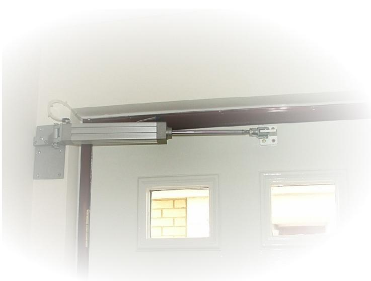
The Radio Frequency Door Opener System will enable you to unlock, open, close and relock your door by remote control using a small battery operated Transmitter.
